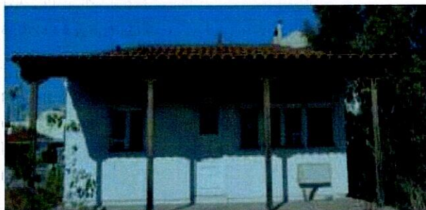
Picture 2: Small Building where the air pollution station is installed
